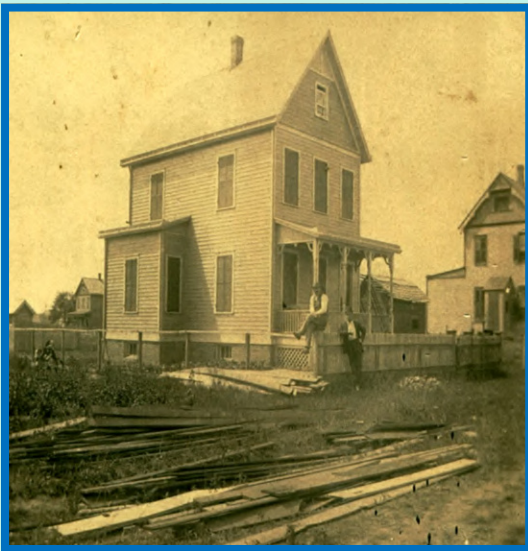
A Peetzburgh house under construction. Each house looked the same and cost about $800. The house had two stories and a front porch. Several dozen of these houses survive today. Most have been updated with modern comforts, but many have retained their period charm.
